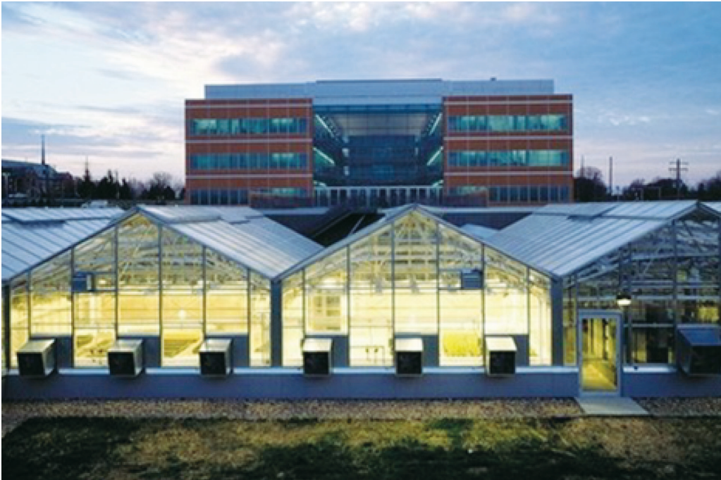
Plant Containment Facility (Source: Emec Technology)
